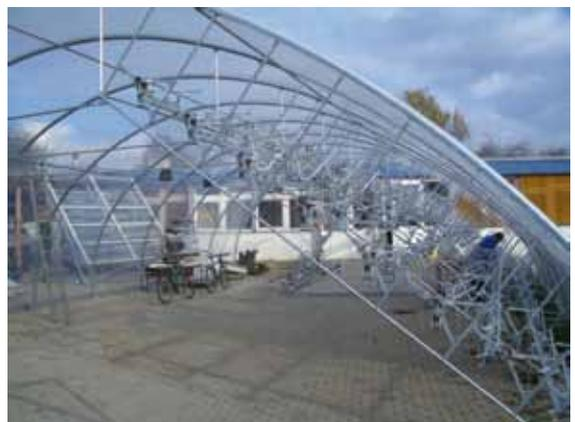
The optical systems, mounted in the roof of the greenhouse are protected from wind and weather, are designed extremely light and inexpensive.
